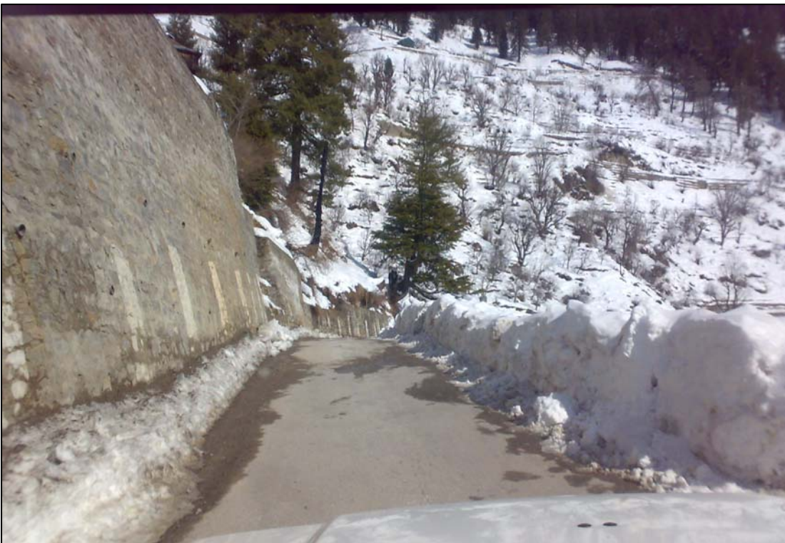
D-16: A view of road constructed along Allain stream
