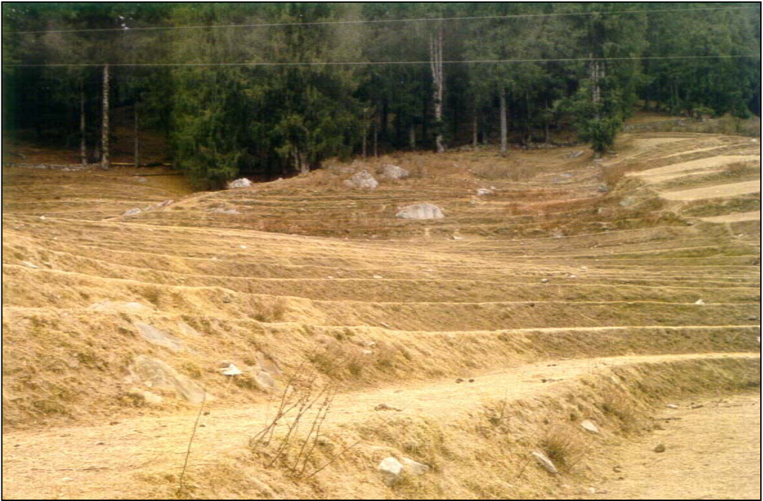
Figure D-5: View of the terraced land at proposed Forebay reservoir
